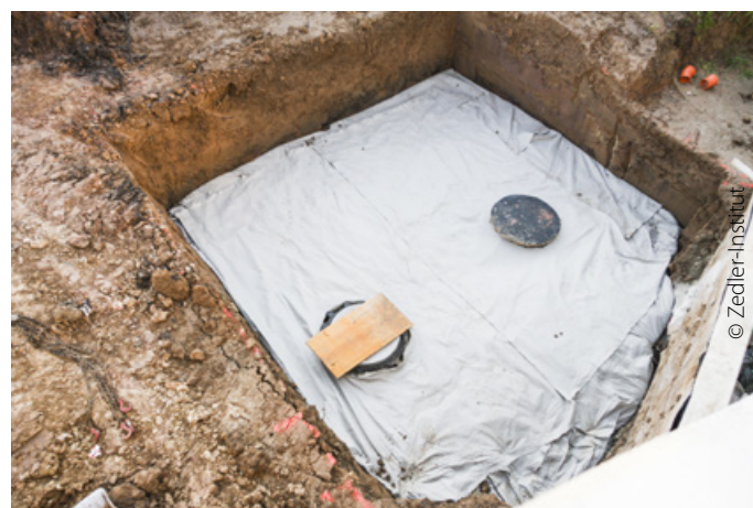
Rain water cistern after installation
