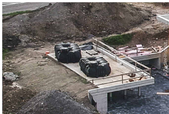
Rain water cistern (two times 5,000 l) prior to installation
